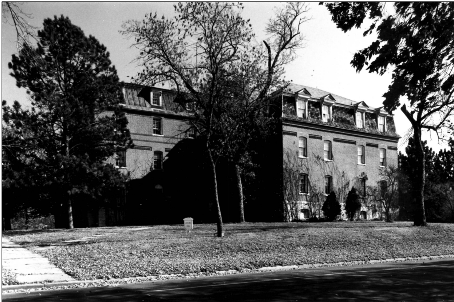
Photo 2 – west elevations of Gaylord Hall showing the west wing at right, looking ESE Photo by David Murphy, 1975, NSHS (7510/1:3)
